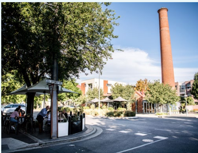
Former City Destructor Complex Heritage Adaption
